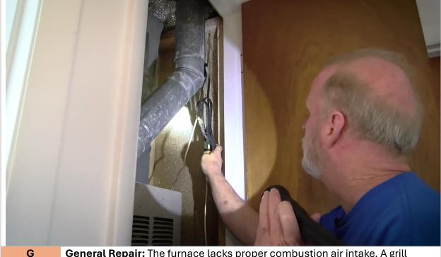
**General Repair:** The furnace lacks proper combustion air intake. A grill should be installed on the door to allow for adequate air flow.
