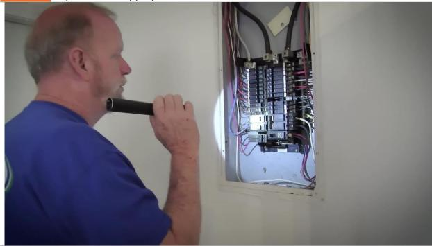
**Functional:** The main electrical panel is accessible and in generally good condition. No signs of overheating were detected during the thermal scan of the breakers.
